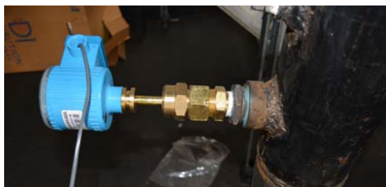
Figure 4-81. Glycol loop insertion style flow meter.
