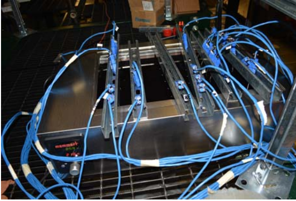
Figure 4-82. Thermocouple oil bath front view.
