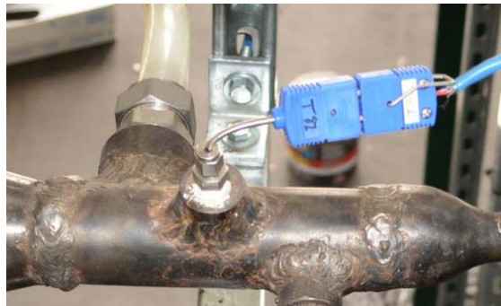
Figure 4-73. Thermocouple in pipe.
