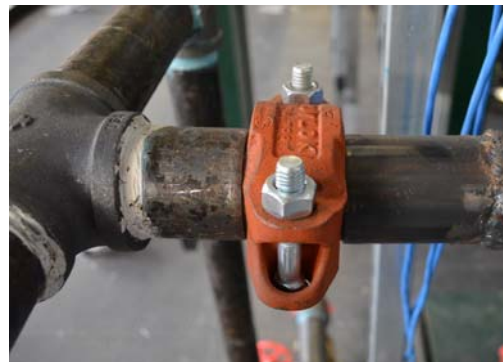
Figure 4-49. Grooved connection.
