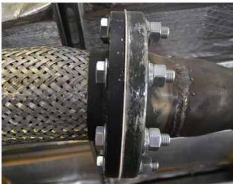
Figure 4-48. Flanged connection.
