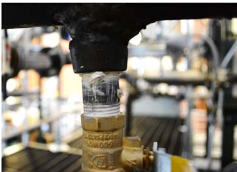
Figure 4-50. Threaded connection.
